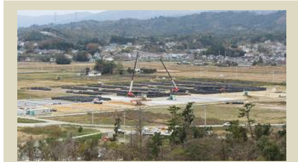
Construction of a temporary storage facility for decontamination waste
