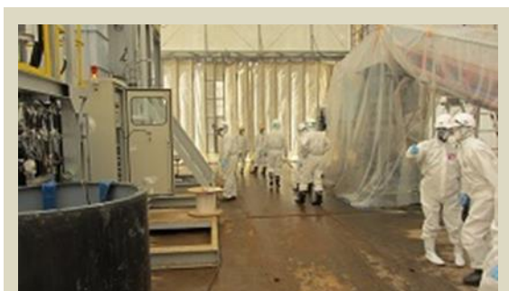
Experiment to test the fixation of designated waste (fly ash) in cement
