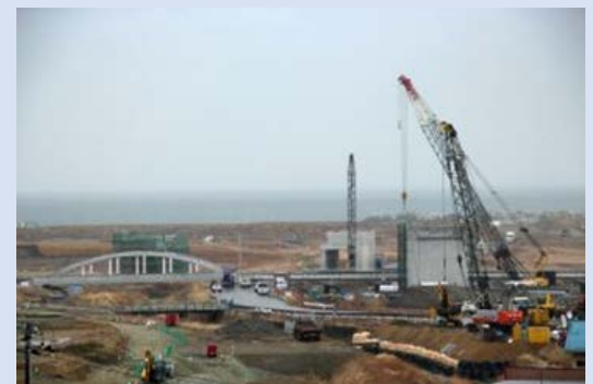
Reconstruction in progress (photo: NPO Miraito)
