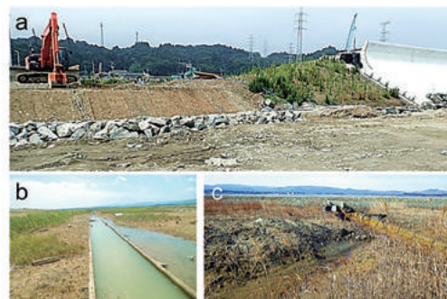
Figure 5. Photo a: Disappearance of the tidal flats as a result of seawall construction in the Same River estuary; Photos b & c: Tidal flat restoration in Ohsu conservation area, Matsukawa-ura (Photo b by Dr. Takahide Kurosawa, Photo c by Dr. Takao Suzuki)
