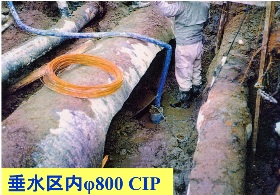
Cast iron pipes (CIP)
