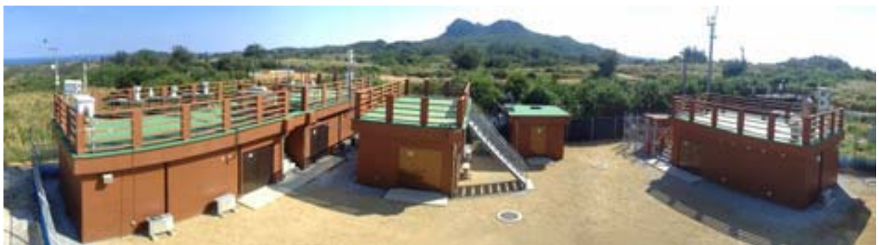
Cape Hedo Aerosol and Atmosphere Monitoring Station (CHAAMS) in Okinawa, Japan
