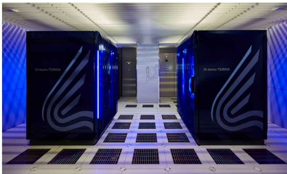
Fig. 1 The NEC SX-Aurora TSUBASA supercomputer
