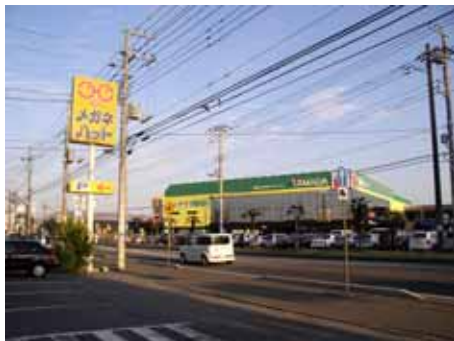
Fig. 7 Shopping area, chaotic electric cables
