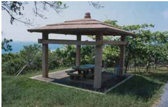
Fig. 1 A picnic shelter in a park in Okinawa where the steep bank between the shelter and path makes it inaccessible for wheelchairs or older people with mobility problems
