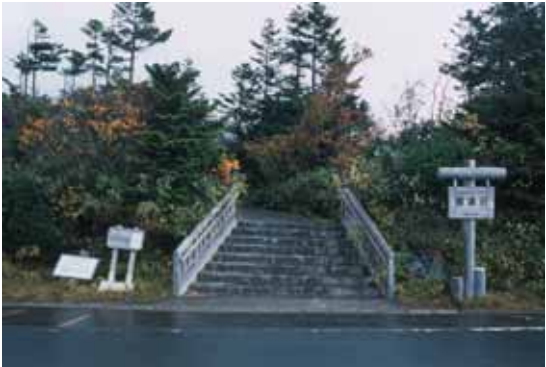
Fig. 4 The entrance to the viewing area which has a flight of steps and no alternative access. This spoils an otherwise exemplary facility
