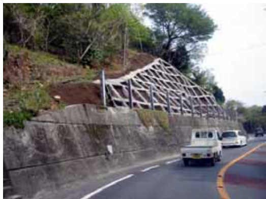
Fig. 14 Slope stabilization through a concrete grid, near Atami
