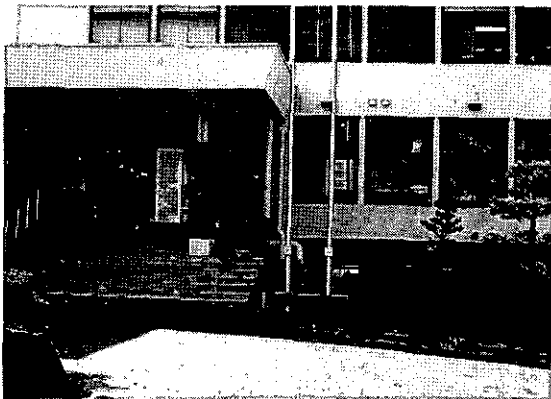
写真 2 抜け上がった福富町役場 (1989年10月には玄関の階段が7段付け加えられていた) Photo.2 Lift up of the Fukutomi town office building due to land subsidence. (In October 1989, seven risers had to be added to the front steps of this building.)
